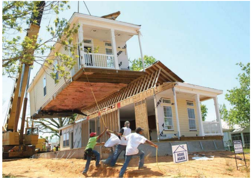
Local residents participate in a houseraising financed by ECDI/Hope Community Credit Union in Mississippi after Hurricane Katrina. The local credit union was instrumental in helping storm victims recover from the disaster.
